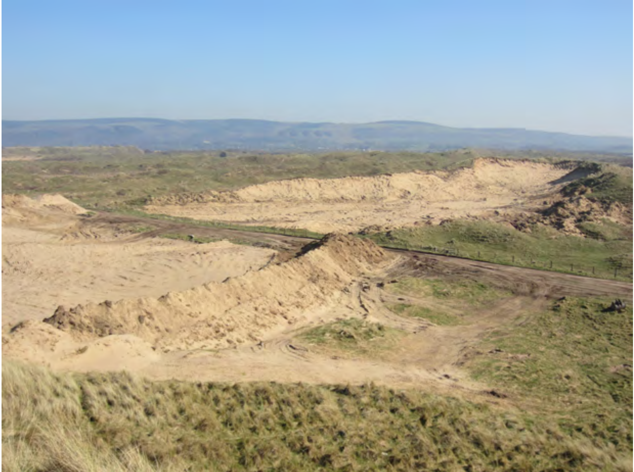
Above and right: Recent excavations at Kenfig sand dunes © Scott Hand, CCW
