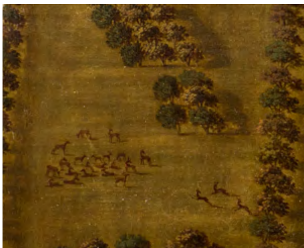
Detail of View of Margam House, Glamorgan, Looking North , c. 1700
