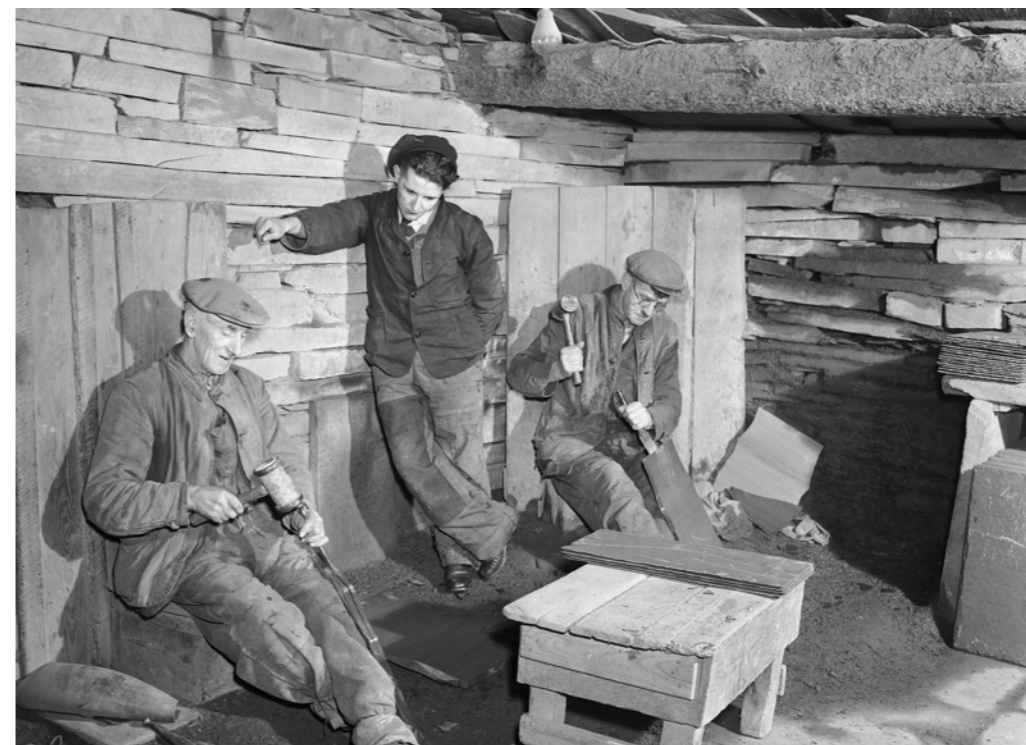
Splitting the slate with a hammer and chisel
