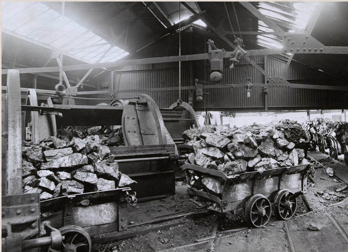
Cambrian coal mine: Electric tipping trams
